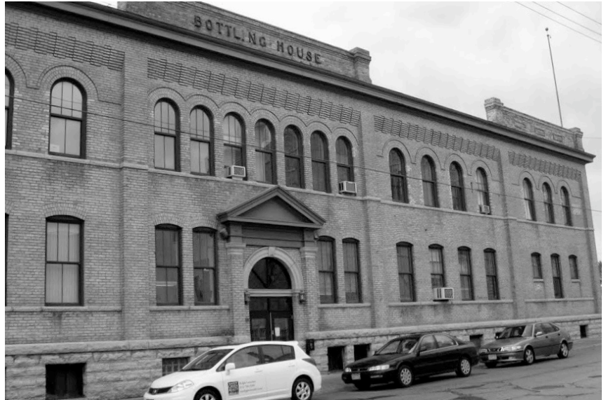
The Grain Belt Bottling House, location of the New IWW offices. Photo courtesy Jeff Pilacinski.
